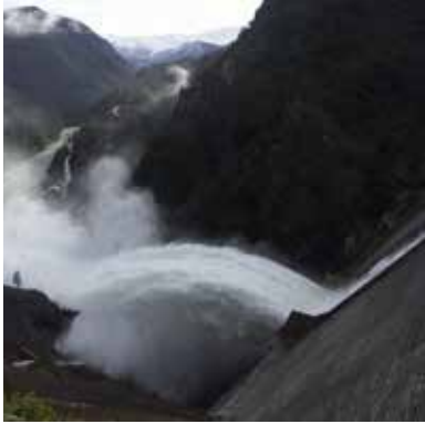
▲ Bio Bio river dam
